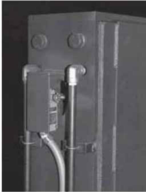
3LS Gate Limit Switch
